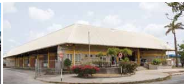
Speightstown Bus Terminal
